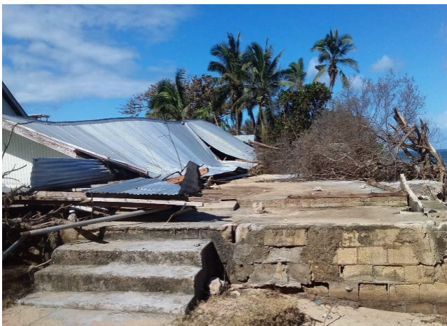
Atata area damage.
