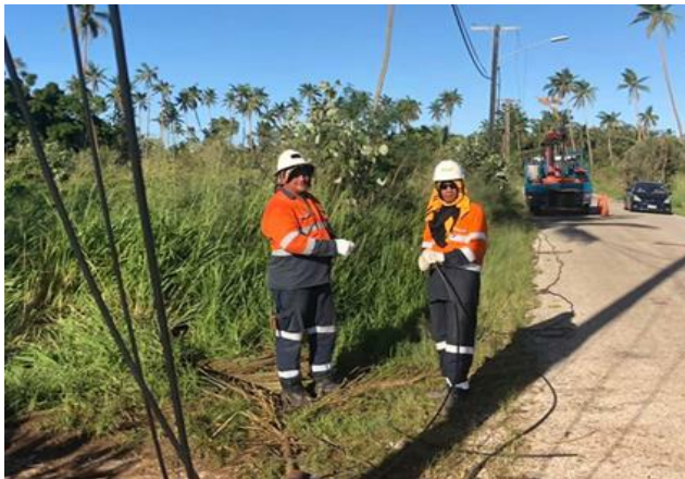
TPL staff members restoring electricity
